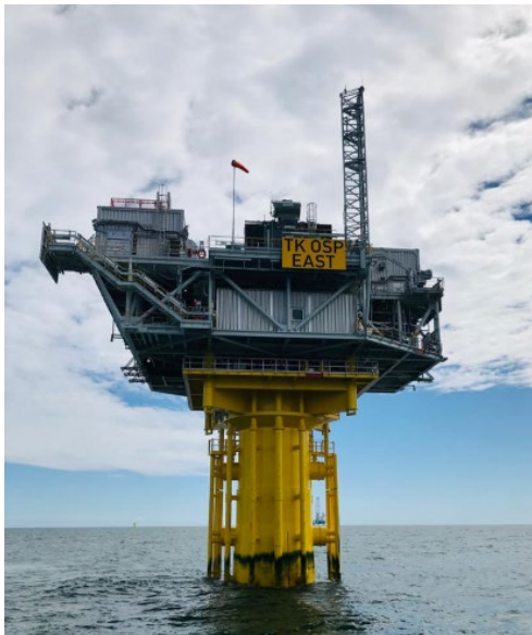
Plate 2.6 Example offshore substation platform (image courtesy of RWE)
