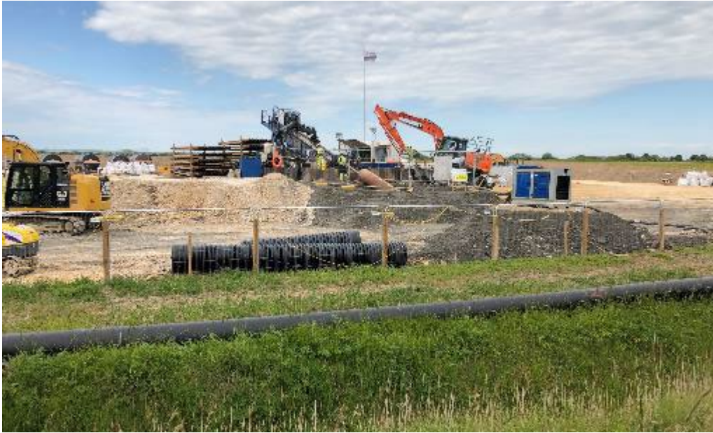
Plate 2.9 Example of a horizontal direction drill rig at landfall – the cable duct is closest in the foreground (image courtesy of RWE Renewables)
