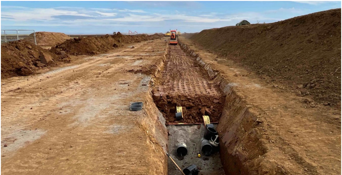
Plate 2.10 Example of a cable trench, once cable ducts have been installed and trench has been backfilled (image courtesy of RWE Renewables)
